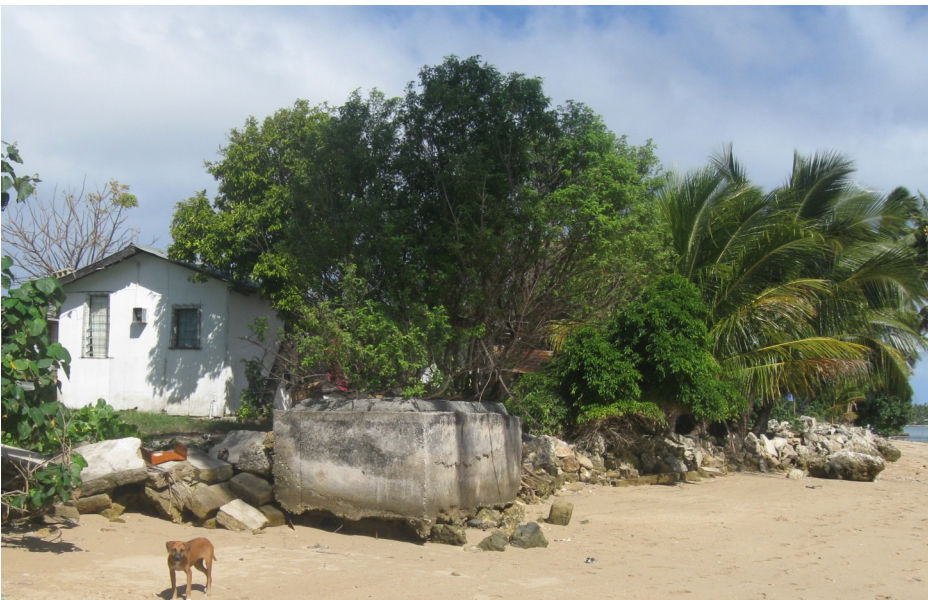
Increasing coastal erosion in Tonga threatens homes
